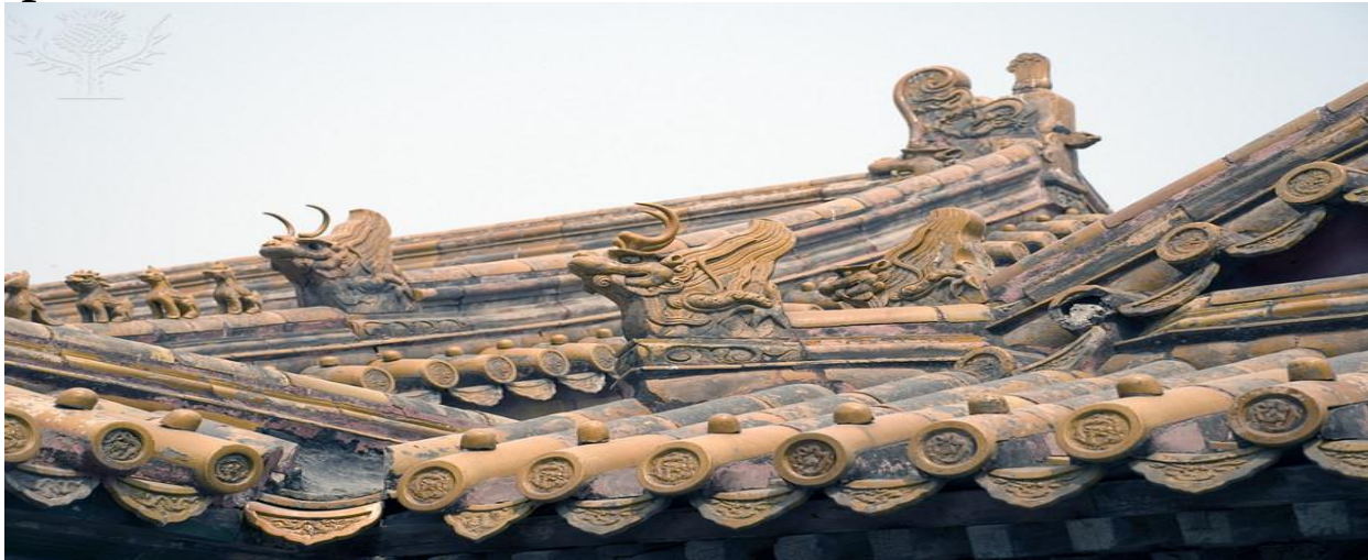
Roof Detail. Photography. Encyclopædia Britannica Image Quest. Web. 26 Feb 2013. http://quest.eb.com/images/131_1871129
